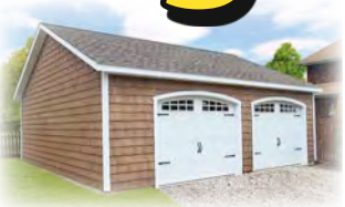
Classic T-111 Built on Site—no floor 7/12 roof pitch
