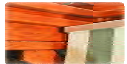
2x2 guide bars ensure that the canopy arms stay level and true.
